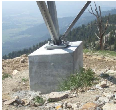
Micropiles Encased in a Pile Cap
