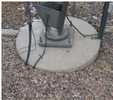
Drilled Shaft at Guy Mast
