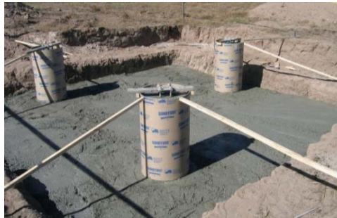
Spread Footer w/ Pedestals
