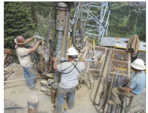
Installation of Micropiles
