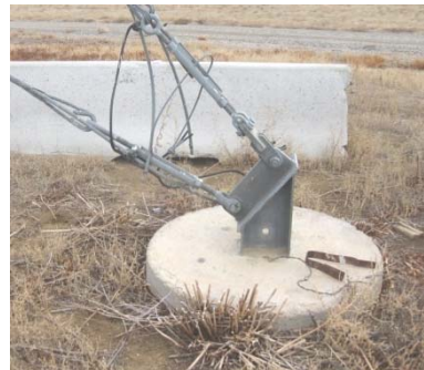
Drilled Shaft at Guy Anchor
